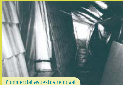
Commercial asbestos removal
